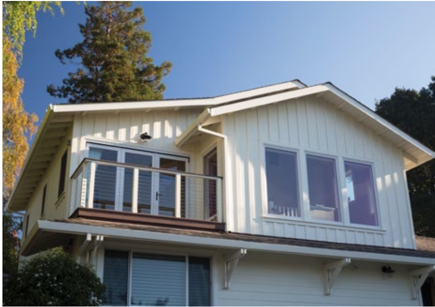
Master bedroom addition with sitting room.
