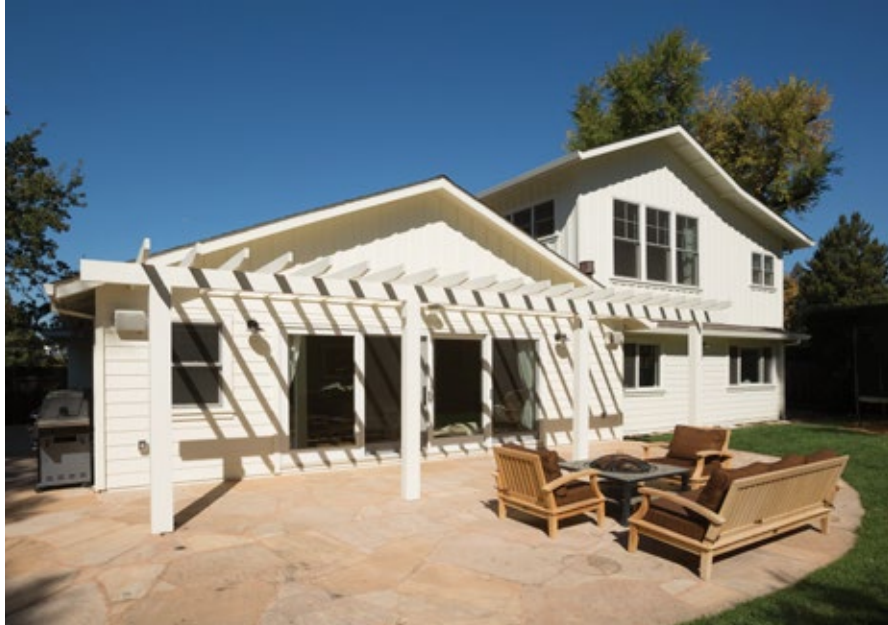
Rear view of master bedroom addition and remodel to living room.
